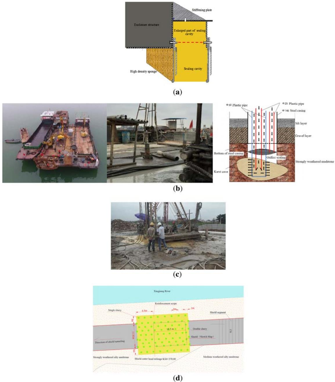
**Figure 10.** Construction risk control measures of Hejiangtao Xiangjiang Tunnel: (a) starting and sealing method of a large slope shield, (b) cyclic static pressure grouting reinforcement technology, (c) reinforcement site of river levee by jet grouting pile and (d) grouting reinforcement at the position of shield machine tool change.
