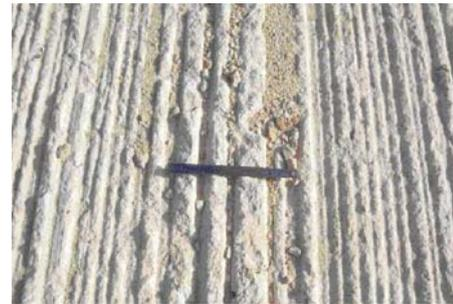
Figure 4. Profile of grooves with spacing of cutting tools.
