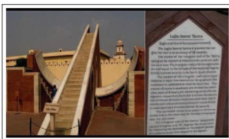
The Samrat Yantra, present in all the Jantar Mantar observatories, is the best known of all the ‘equinoctial’ or ‘equal hour’ sundials in the observatory. Other examples of equal hour time measurements in the observatories are the Nadivalaya Yantra, and time measurement in the bowl of the Jaiprakas Yantra.
