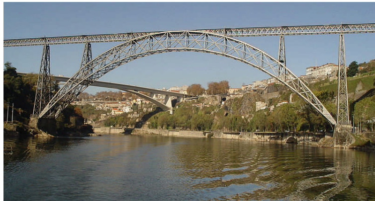
Figure 1. The Maria Pia double hinged arch bridge over the Douro River, Portugal.
