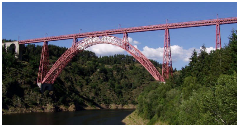
Figure 4. Garabit Viaduct: railroad bridge.
