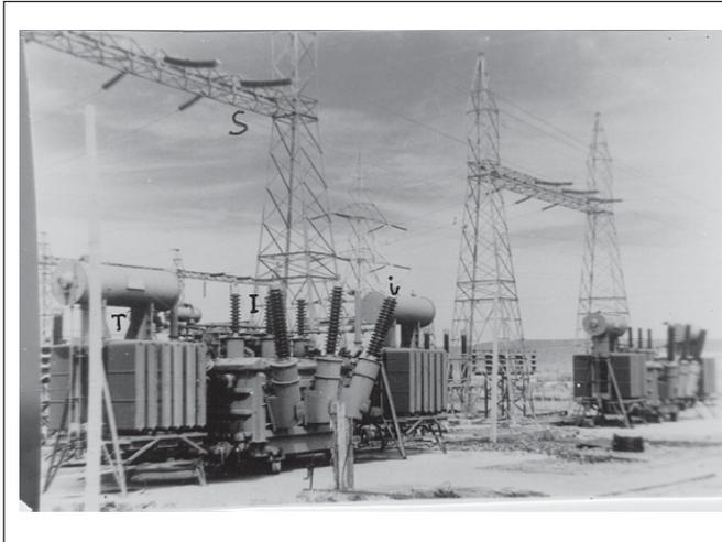
T represents a transformer. The tank placed above it contains oil. The coils of the transformer are wound around a core (made of steel laminations) and immersed in oil which removes the heat produced in the core and the coils.
