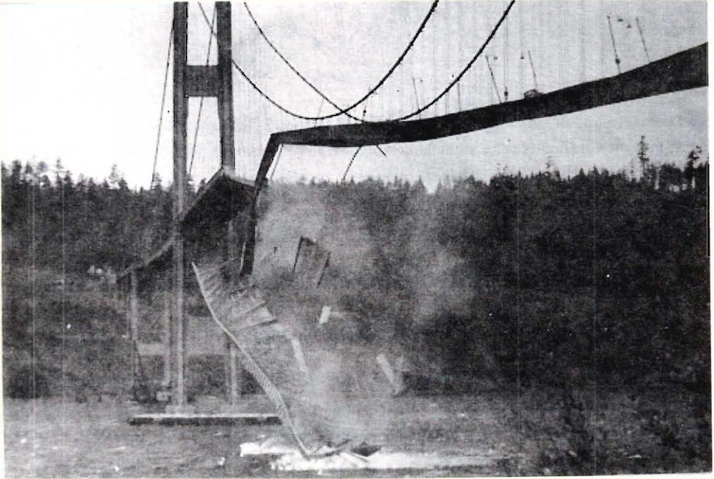
***Caption. Photograph showing the collapse of the Tacoma Narrows Bridge. This photo was taken a few minutes after the first piece of concrete fell, and shows a 600 foot section of the suspension span crashing in to the waters below. A stranded car can be seen on the top right corner. (Picture taken from <http://www.enm.bris.ac.uk/research/nonlinear/tacoma/tacoma.html>)***
