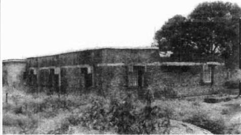
(b) A building with horizontal lintel band in Killari village: no damage
