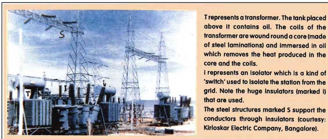
**T** represents a transformer. The tank placed above it contains oil. The coils of the transformer are wound round a core (made of steel laminations) and immersed in oil which removes the heat produced in the core and the coils.
