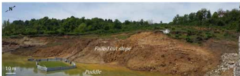
Figure 2. Field view of the Ulubey landslide.
