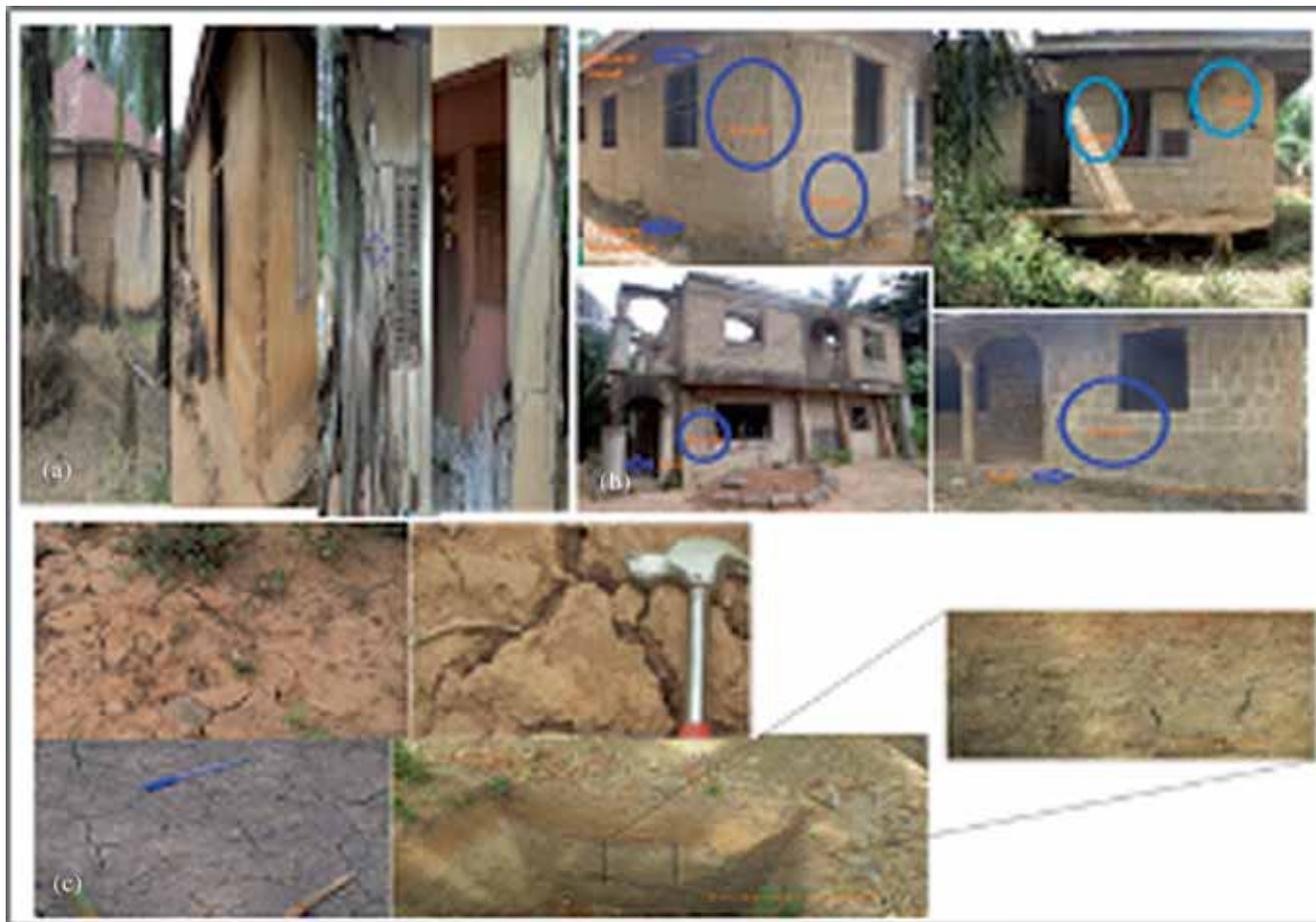
Figure 2. Evidences of expansive soils.
