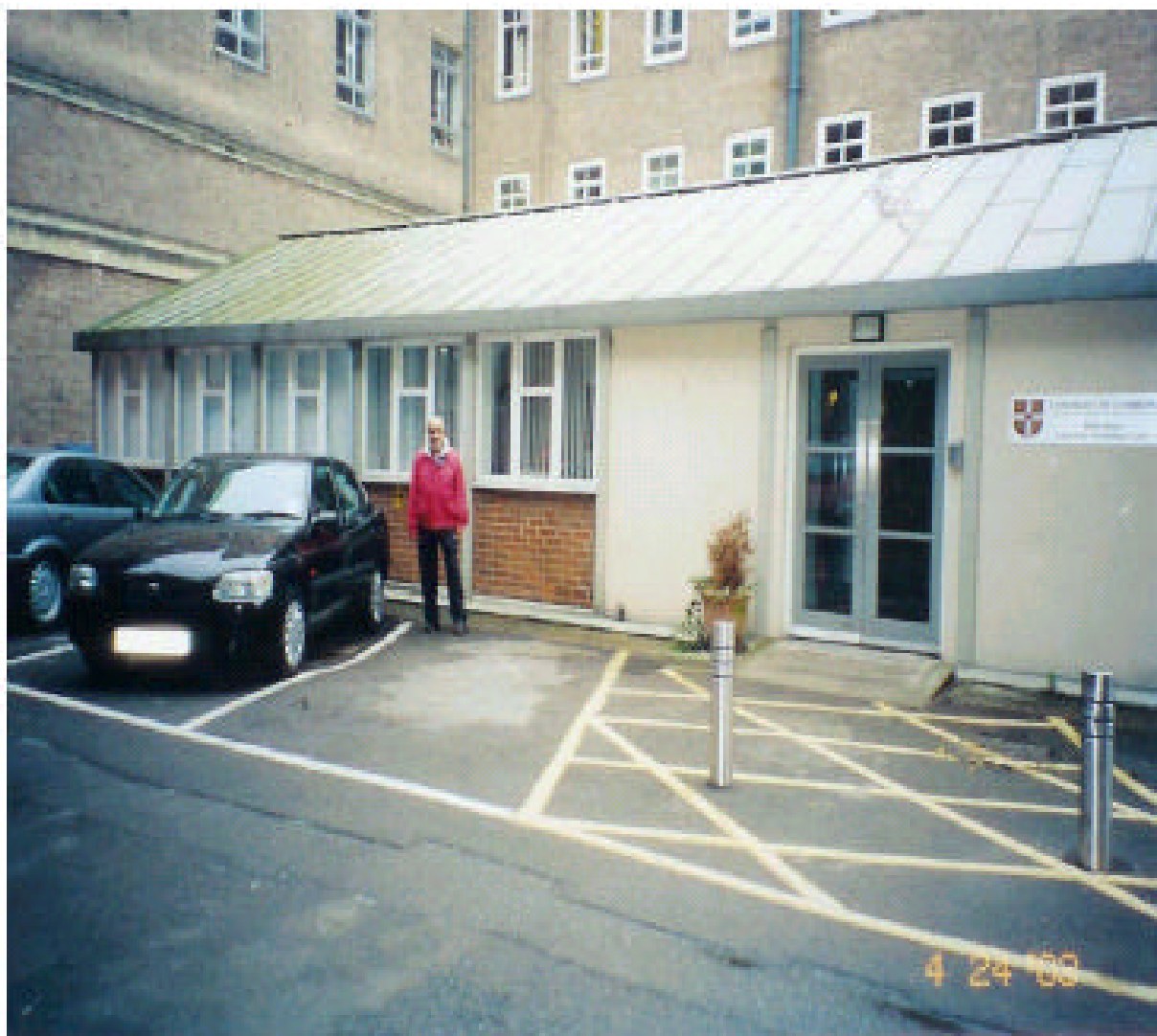
Figure 1. The old MRC prefab building (photograph taken in 2003).
