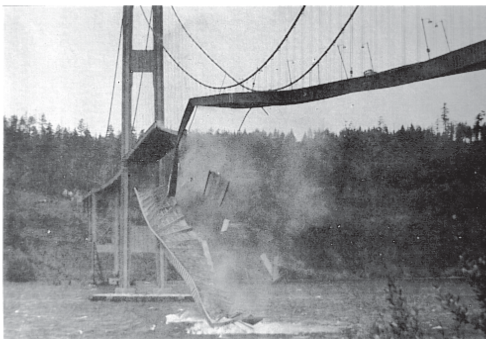
Caption. Photograph showing the collapse of the Tacoma Narrows Bridge. This photo was taken a few minutes after the first piece of concrete fell, and shows a 600 foot section of the suspension span crashing in to the waters below. A stranded car can be seen on the top right corner. (Picture taken from http://www.enm.bris.ac.uk/research/nonlinear/tacoma/tacoma.html )
