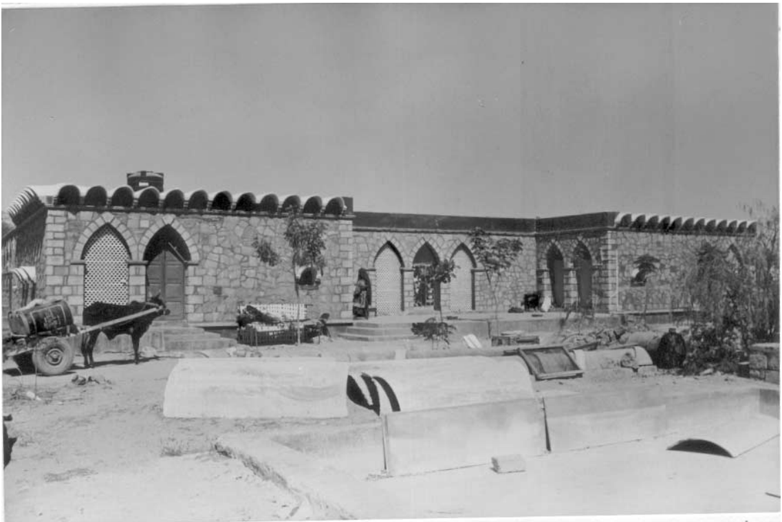
Figure 8. Well dressed stone in CM with ferrocement roof (Khavda).
