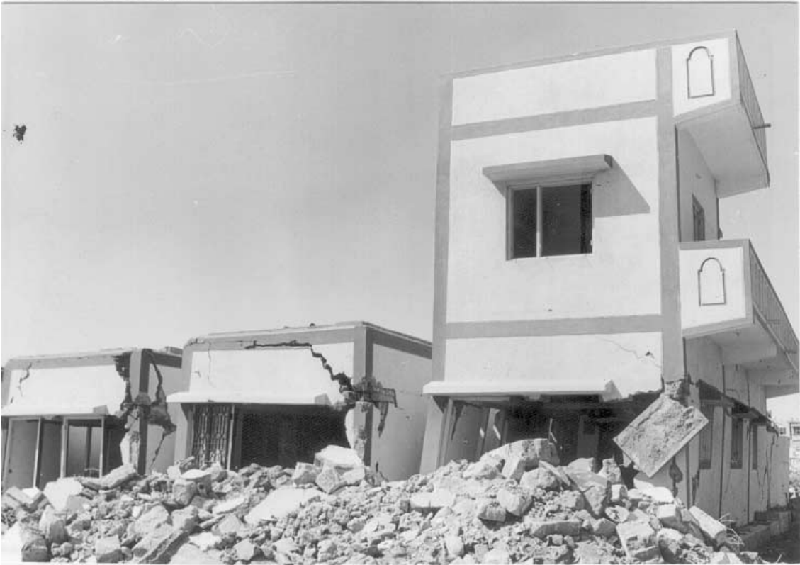
Figure 11. Rigid box-like behaviour above lintel band (Bachau).
