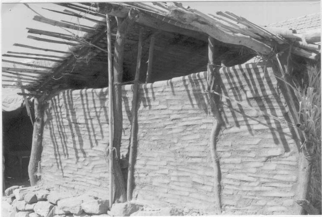
Figure 9. 'Naliyawali Deewal' (Jhadawas, Rapar taluk).
