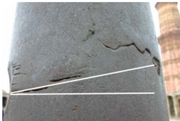
Figure 6. Cracks on the right side of the cannon shot indentation area are aligned in the direction of propagation of the shock wave generated due to the impact (slanted line).
