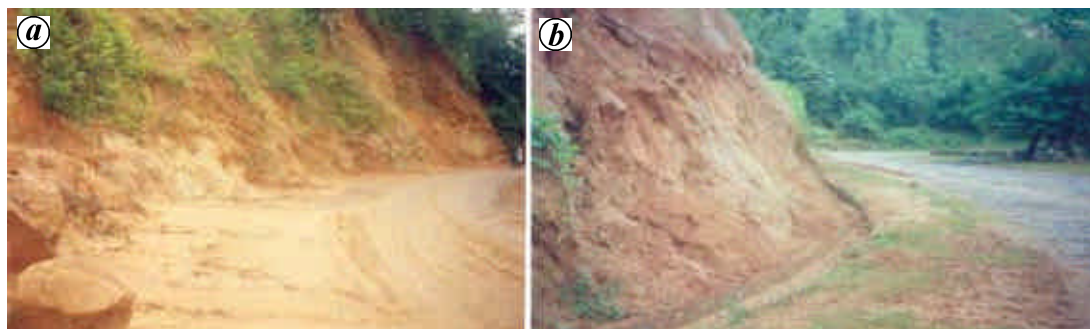
Figure 1 a, b. Ferns and other important plants sliding down with huge forest soil due to road-cutting.
